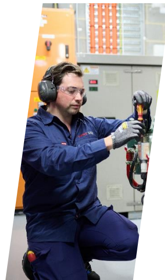
664,105 Reactive Jobs Completed
